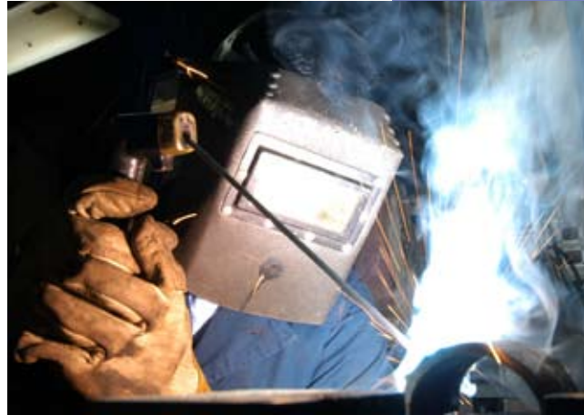
Shielded metal arc welding
